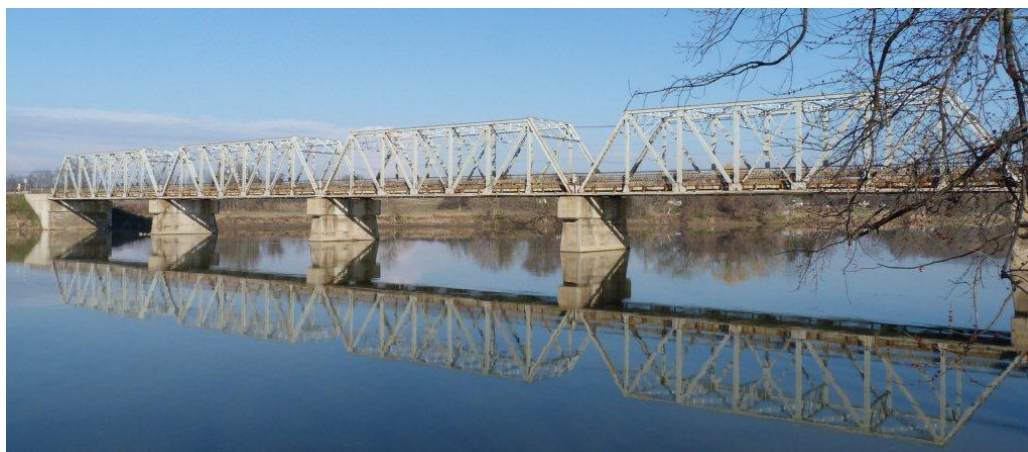
Figure C.10.1 Highway 3 Grand River Bridge Current Condition
